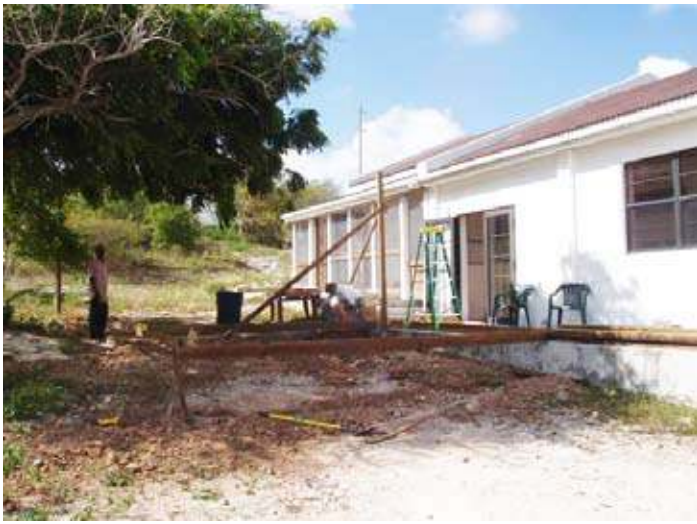
Before and after the work on the second visit. On the left, Judnel and Mary clear drainage, level the ground (as much as possible), glean gravel and set the level frame for the new decking. In both pictures, the accommodation part of the building is on the left and the display area on the right. In the right picture, the new veranda is nearly complete on the new decking. Looking through it, the infamous laundry and public washroom building can be seen a little way away.
