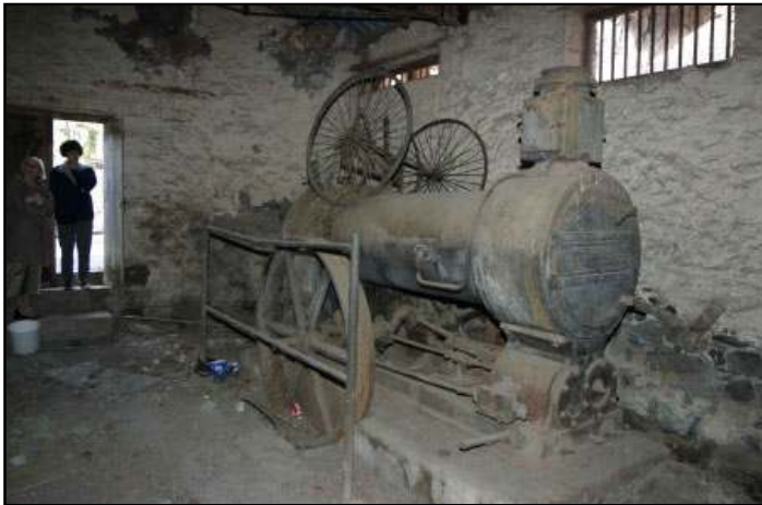
Inspecting the historic building and steam engine that will form key parts of St Helena's flax museum.
