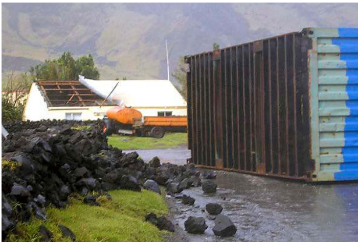
An upturned container, wall collapse (these black boulders are black lava blocks from the 1961 volcanic eruption, used widely for wall-making in the village) and the damaged Government Guest House behind.
