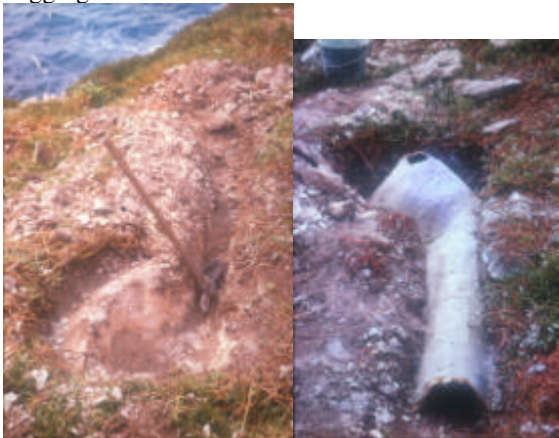
Partly completed concrete burrow
