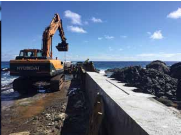
Alternative harbour project: construction of the protective sea wall © Andrew Christian
