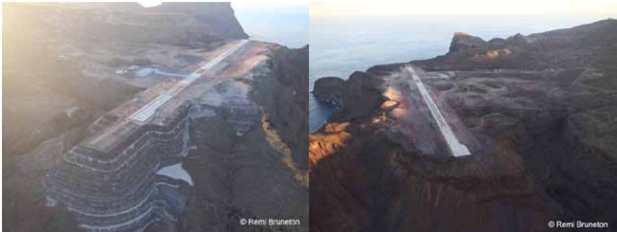
St Helena Airport: aerial views, May 2015
