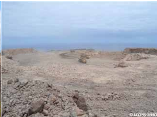
Prosperous Bay Plain during construction
