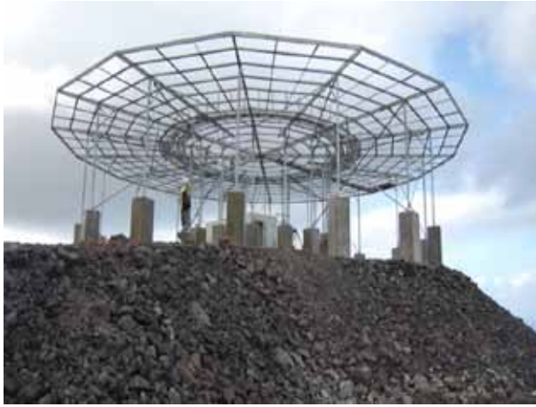
St Helena Airport DVOR under construction at Bradleys
