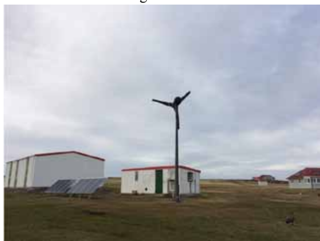
Individual farms are run off-grid. They range from small one-property to larger micro-grid systems. Pre-1996 diesel generators were widely used running for 8 hours per day. After the introduction of a rural energy grant, 24-hour electricity became a possibility, wind hybrid systems and other technologies have been used.
