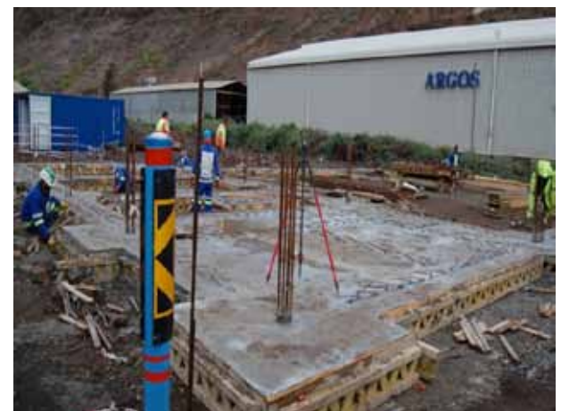
St Helena Airport Sea Rescue facility under construction
