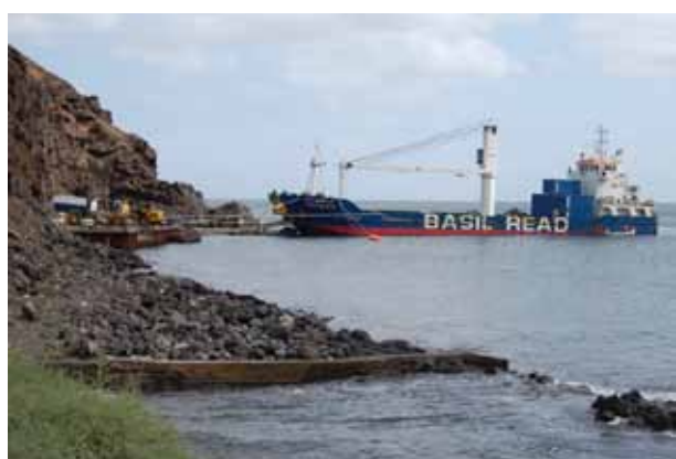
St Helena Airport temporary jetty at Ruperts
