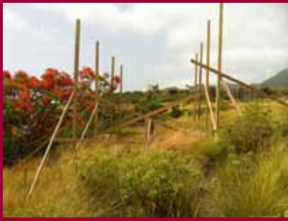
The early stages of construction of Mr Kirnon's model farm. Photo: Andy Kirnon
