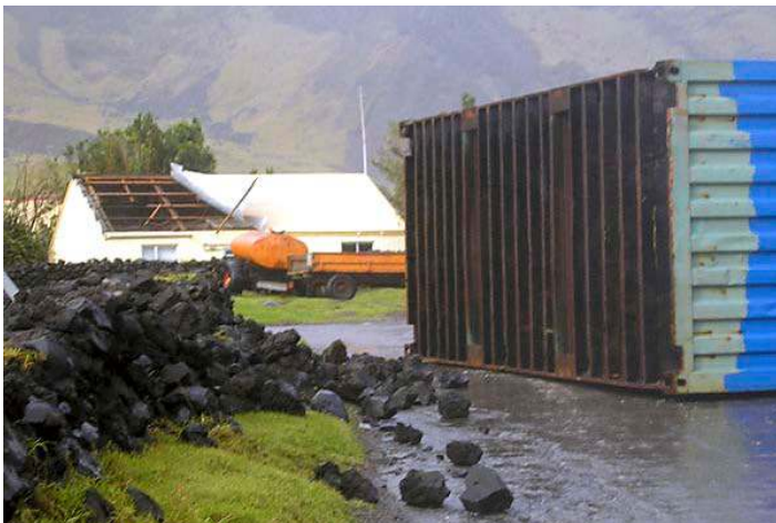
An upturned container, wall collapse (these black boulders are black lava blocks from the 1961 volcanic eruption, used widely for wall-making in the village) and the damaged Government Guest House behind. Photo: Lorraine Repetto
