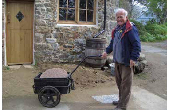
Richard at work on the conservation of the Cider Barn
