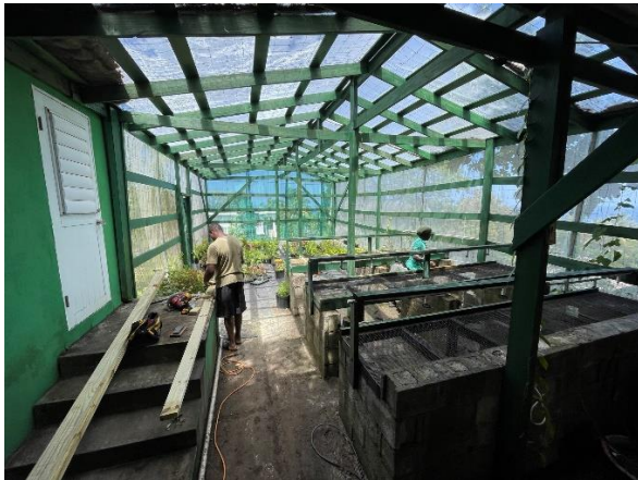
Figure 3 (left): Propagation greenhouse at Montserrat National Trust. The three mist benches on the right side are cleared of plants in this photo as they are having extra wood added to level up the wire on the benches.
