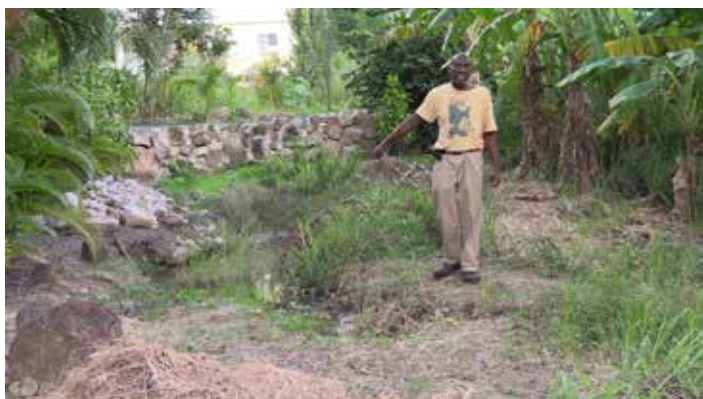
Below: Norman is excavating ponds to help with water control.
