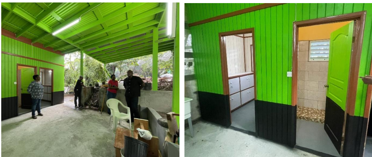
Figure 32: The new covered area and showers/toilets/locker rooms in the MNT nursery.
